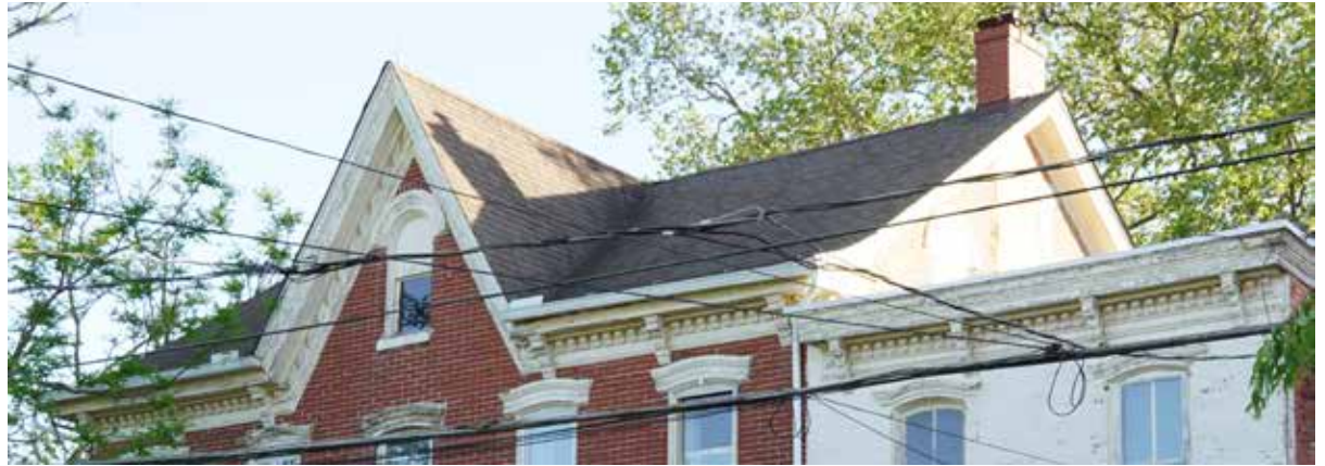
Decorative cornices and lintels along adjacent buildings on Main Street
