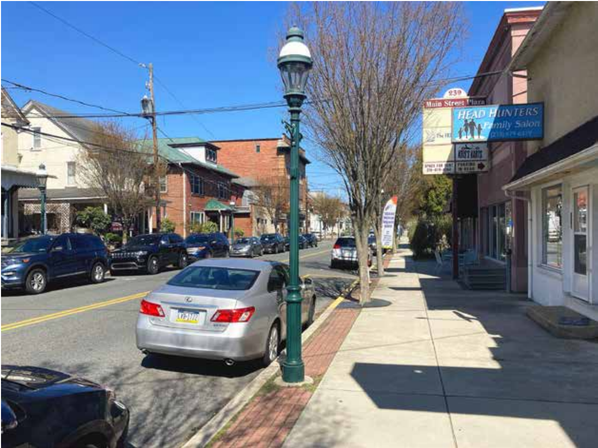
This section of Main Street features brick pavers and a deeper sidewalk than average.
