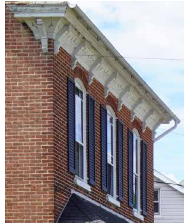
This building has retained the original cornice and window openings
