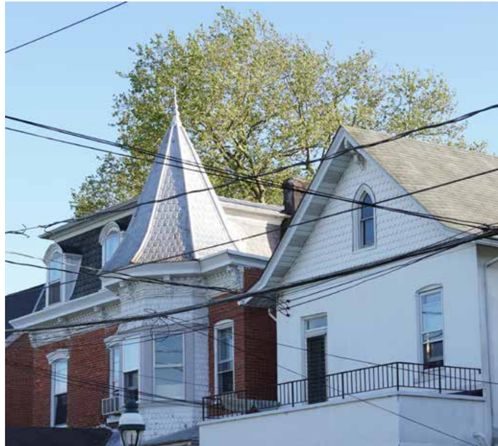
Examples of various roof styles found on Main Street
