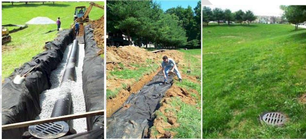
Figure 3: Example of Infiltration Trench Installation
