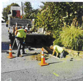
Stormwater Inlet Cleaning
