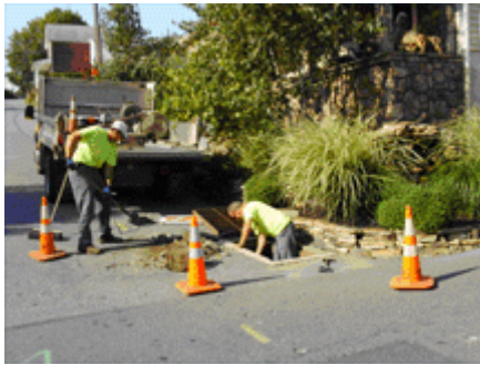
Stormwater Inlet Repairs
