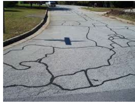
Crack Sealing – Roadway Maintenance
