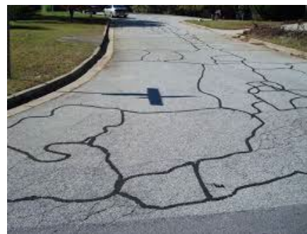
Crack Sealing – Roadway Maintenance
