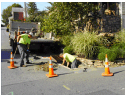
Stormwater Inlet Repairs
