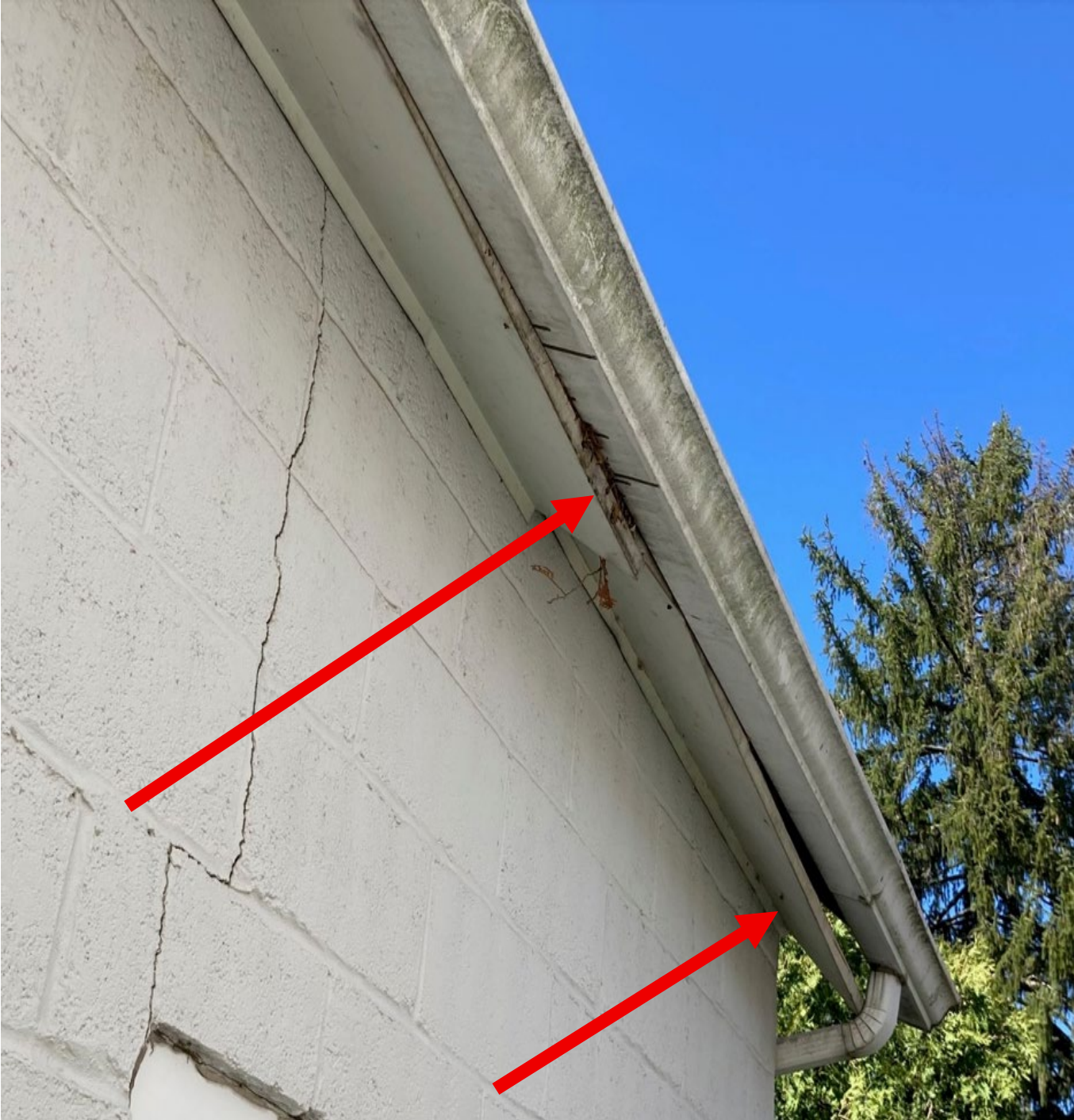
107 N. Fourth St. – Emergency Roof Repair due to rodent infestation
