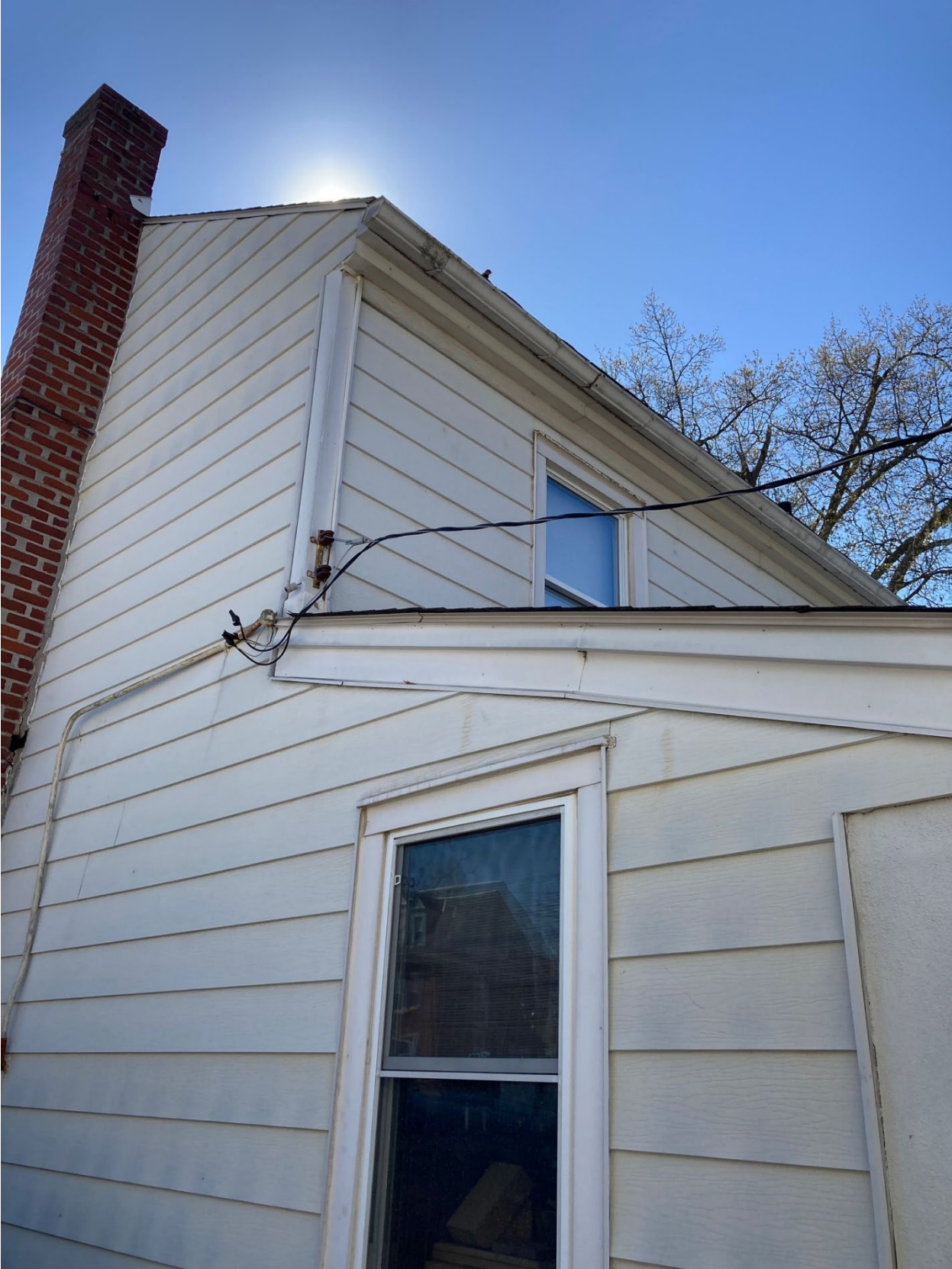
107 N. Fourth St. – Emergency Roof Repair due to rodent infestation
