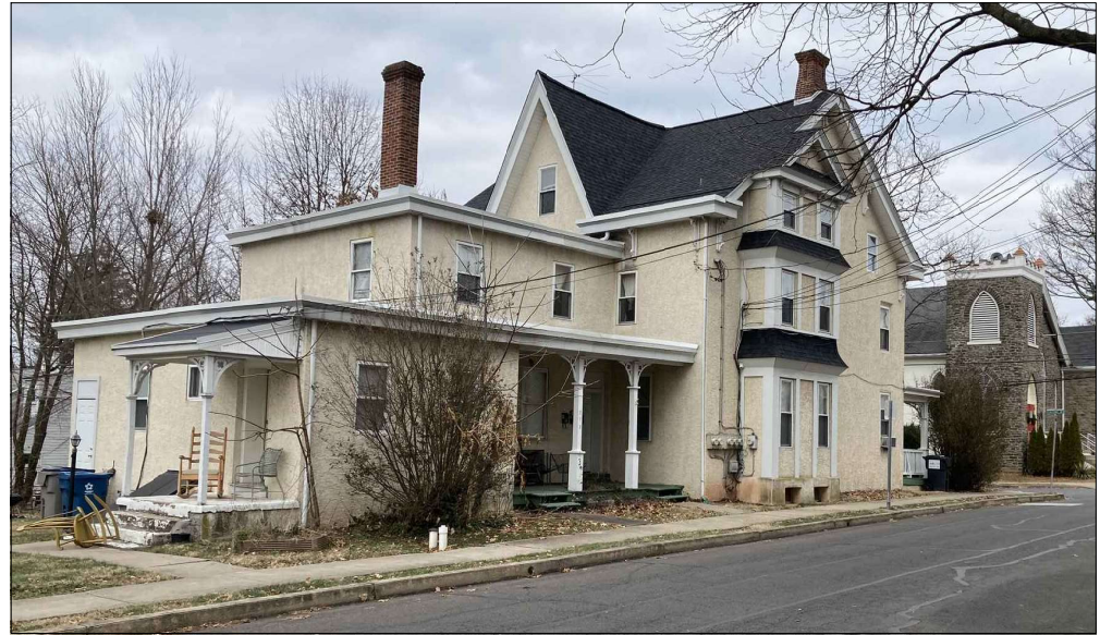
View from Shearer Street - Existing Side Porches
