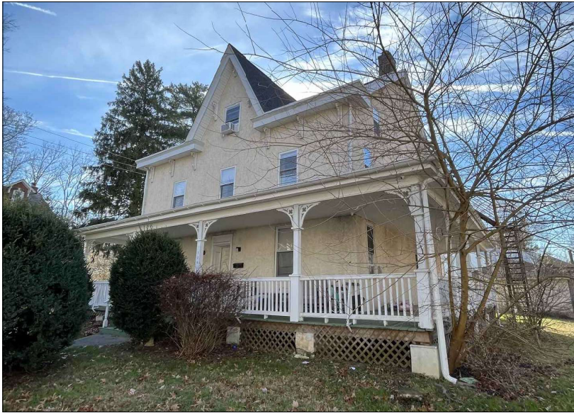
126 S. Pennsylvania Avenue - Existing Front Porch
