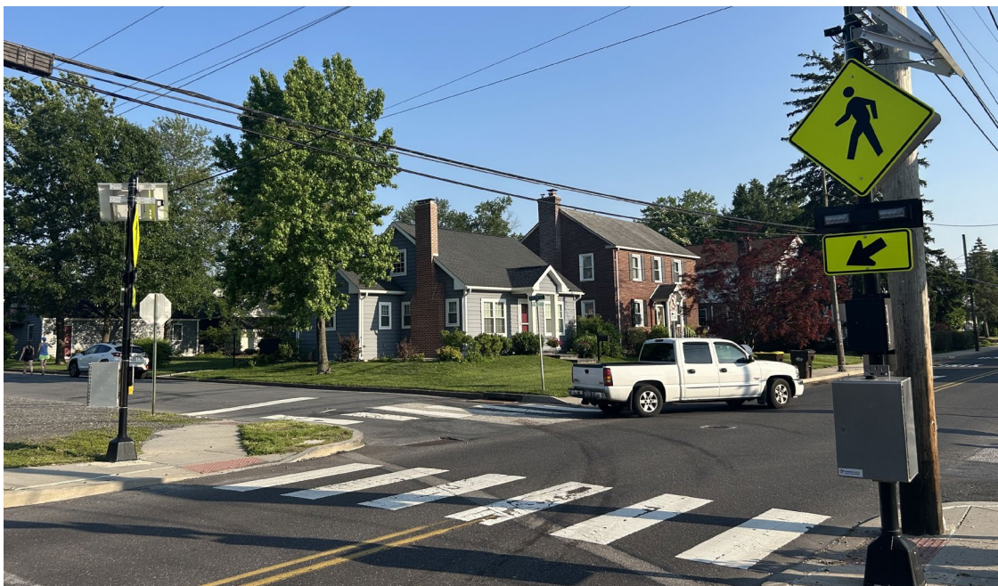
The new pedestrian-activated Rectangular Rapid Flashing Beacon (RRFB) enhances safety for those seeking to cross Walnut Street
