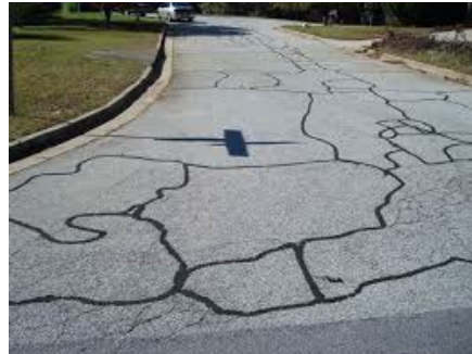
Crack Sealing – Roadway Maintenance
