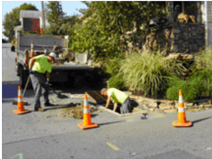
Stormwater Inlet Repairs
