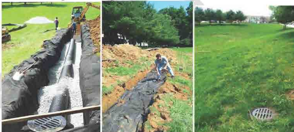
Figure 3: Example of Infiltration Trench Installation
